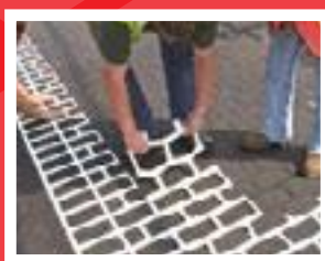
3. DuraTherm™ thermoplastic grid is inlaid into the asphalt.
