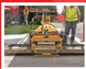
1. Asphalt is heated by the infra-red heater.
