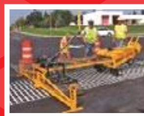
4. Custom-formulated DuraTherm™ thermoplastic is melted in place using the heater.
