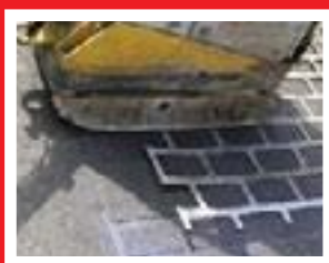
2. DuraTherm™ templates are pressed into the asphalt and then removed.
